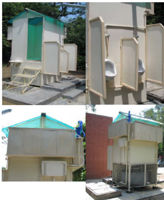
Figure 13: Portable zero discharged toilet system, IIT Kanpur campus
