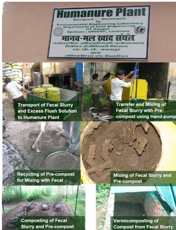
Figure 31: Pictorial representation of transport of fecal slurry and various operations at Humaure Plant
